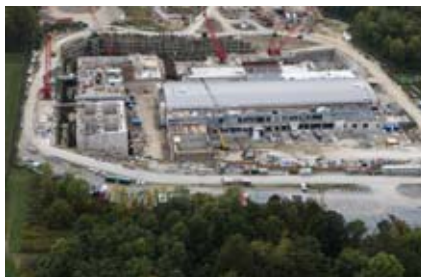
UV plant construction in 2010.
